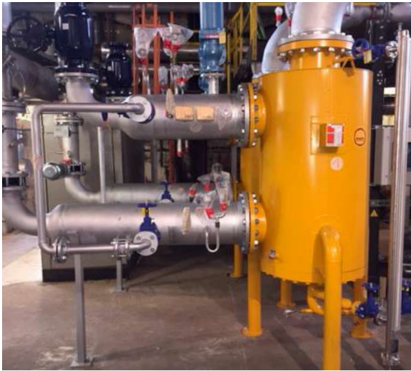
Closed steam heat transfer stations installed for an international stainless steel manufacturer
