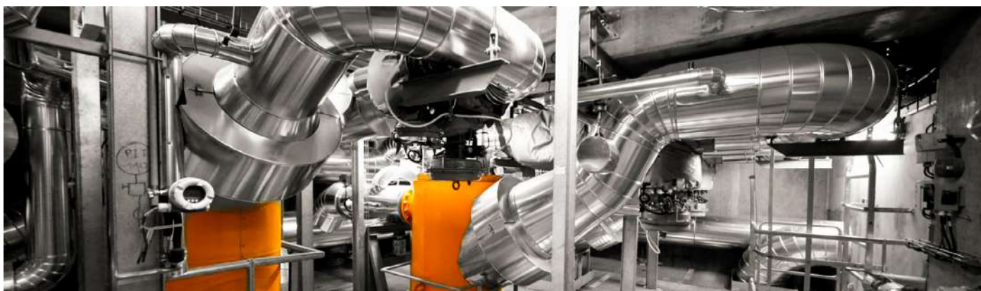
Steam transfer station; Palais Bourbon, Paris
